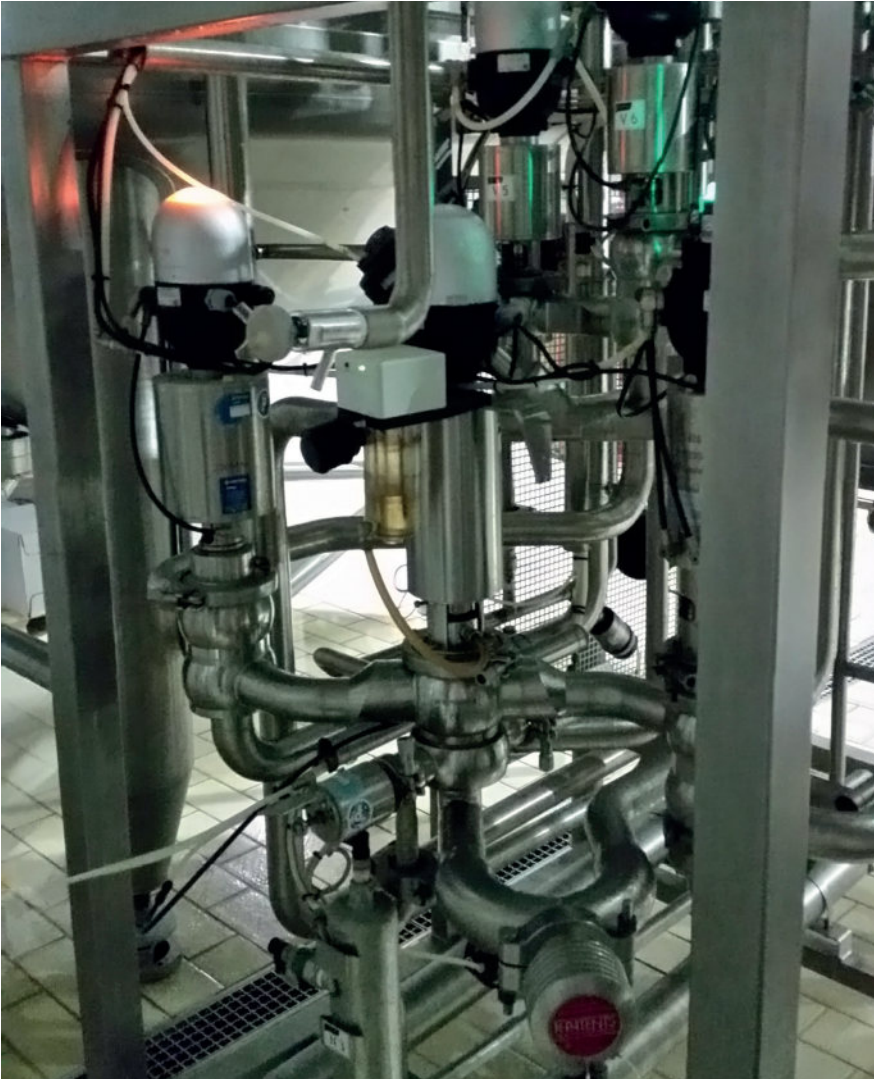
Controlling product flow based on Brix levels, using a combination of a 3 way valve and a Brix meter.
