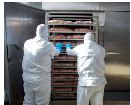
Lutetia® Defrosting chambers
