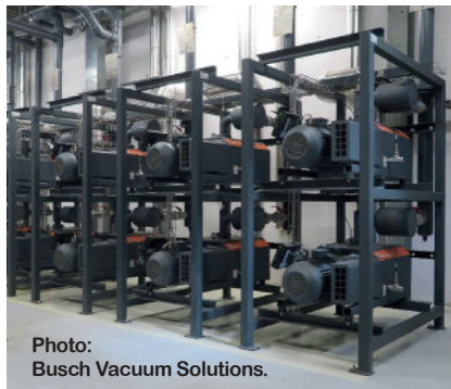
A vacuum system from Busch Vacuum Solutions provides Emsland Frischgeflügel GmbH's transport system with the required vacuum.
