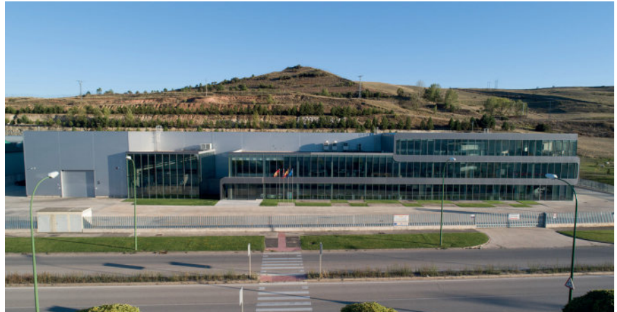
Hiperbaric's Facilities in Burgos, Spain
